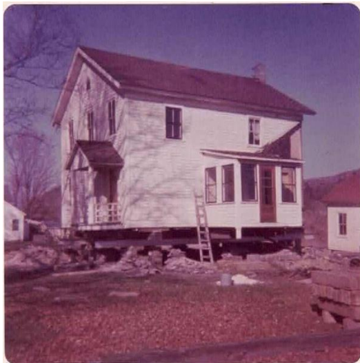
312 Main Street House moving
